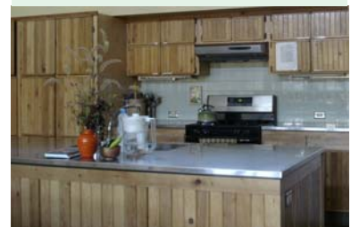
Cabinetry and wainscoting were constructed by students using oak (downstairs) that was recovered from old farm fences on campus and pine (upstairs) from the deconstructed Early Learning center.
