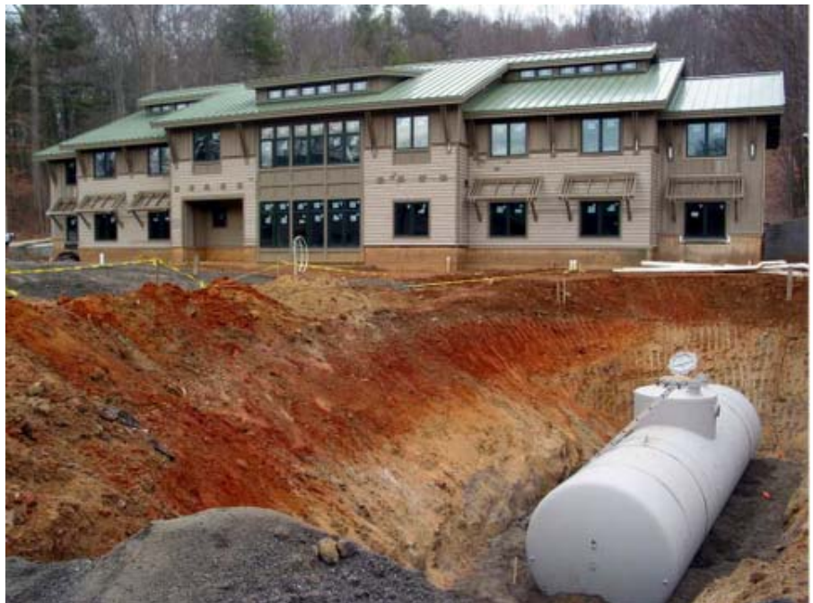
Rainwater is collected in a salvaged milk train car buried in the front yard
