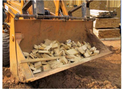
During construction of the EcoDorm, approximately 2,000 pounds of waste was diverted from the landfill.
