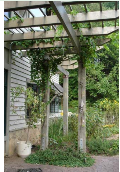
Beams for the trellis and stair supports are salvaged steel
