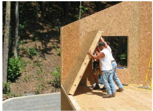
Structurally Insulated Panels (SIPs) can reduce energy costs by 50 percent or more, and are also recyclable.
