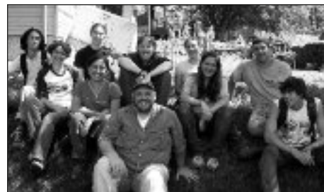
WWC students and ELC staff Phillip Gibson insulate first house.
