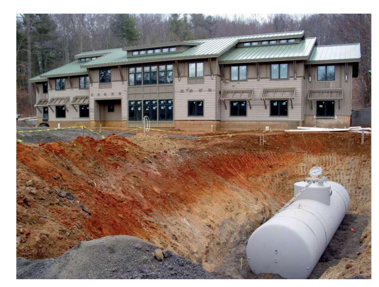
A 10,000 gallon salvaged train tanker car holds rainwater from the roof before it is pumped into the dorm, pressurized, and used to flush toilets, as well as to irrigate the garden
