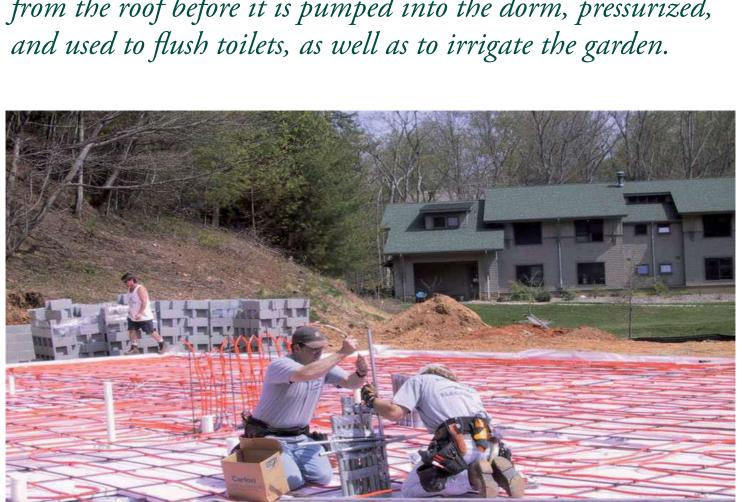
Workers install the hydromatic (radiant hot water) floor heat system. The water is preheated in a solar collector, reducing the energy cost by half.
