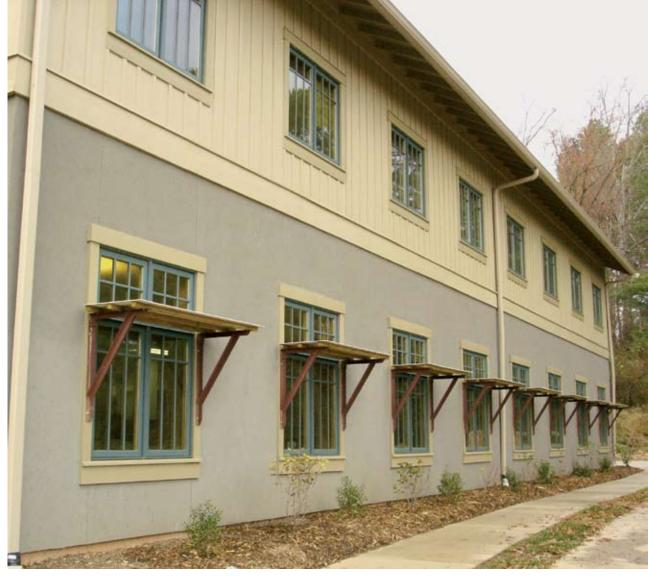
Light shelves reflect sunlight onto interior ceilings to illuminate the offices without glare.
